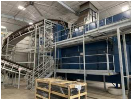
Figure 9: Norris Thermal Technologies pasteurization building used by Merrell Bros (Merrell 2019).
